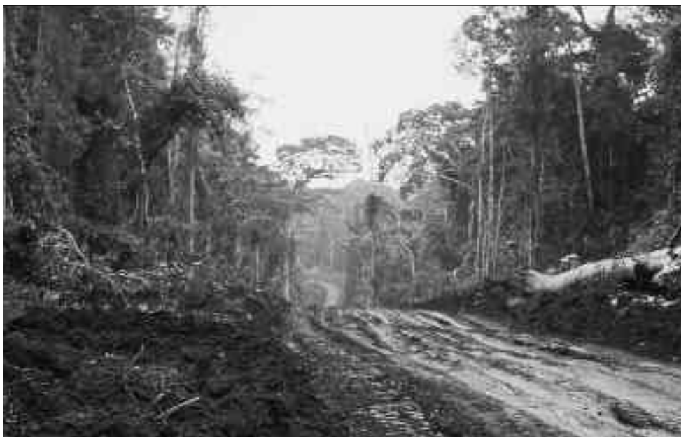
July 2001: new logging road in East Cameroon
